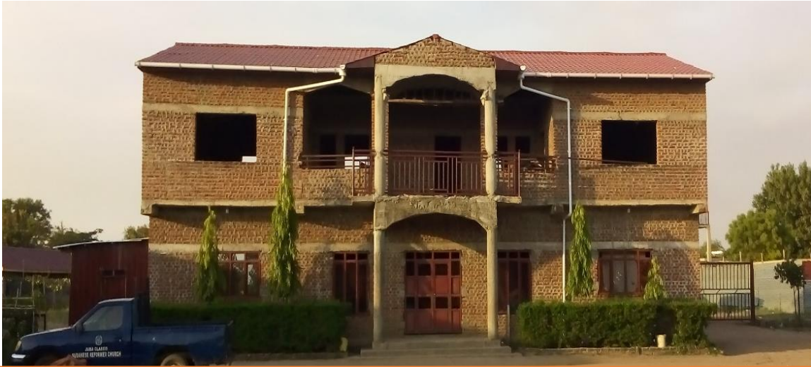
SRC General Synod building under construction
