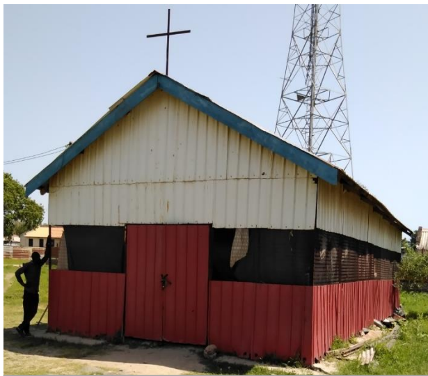
Immanuel SRC church building, Malakal
