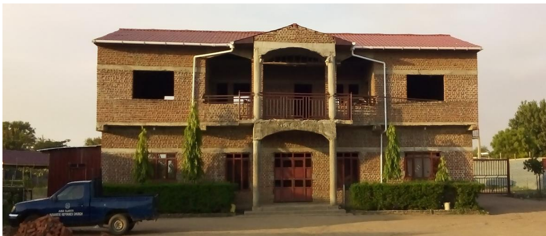
Incomplete SRC Synod building Juba, South Sudan
