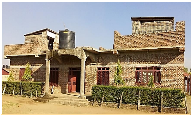
Construction being resumed SRC Synod office, Juba, South Sudan
